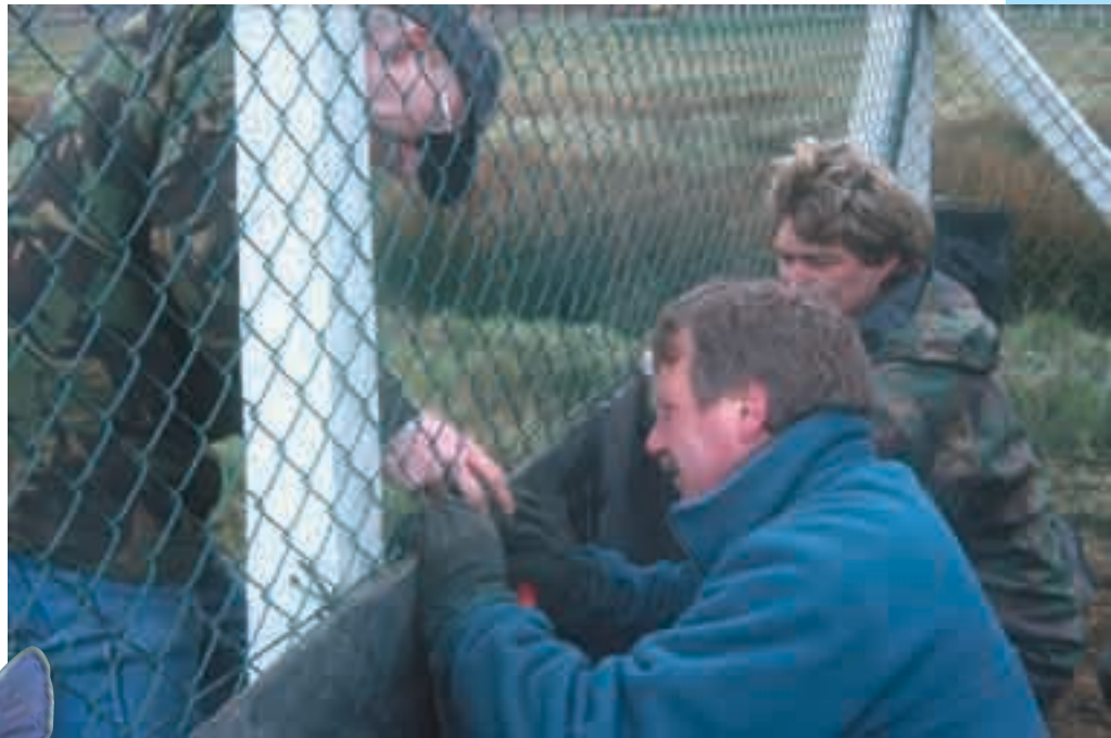
Top Erecting Newt Fence
